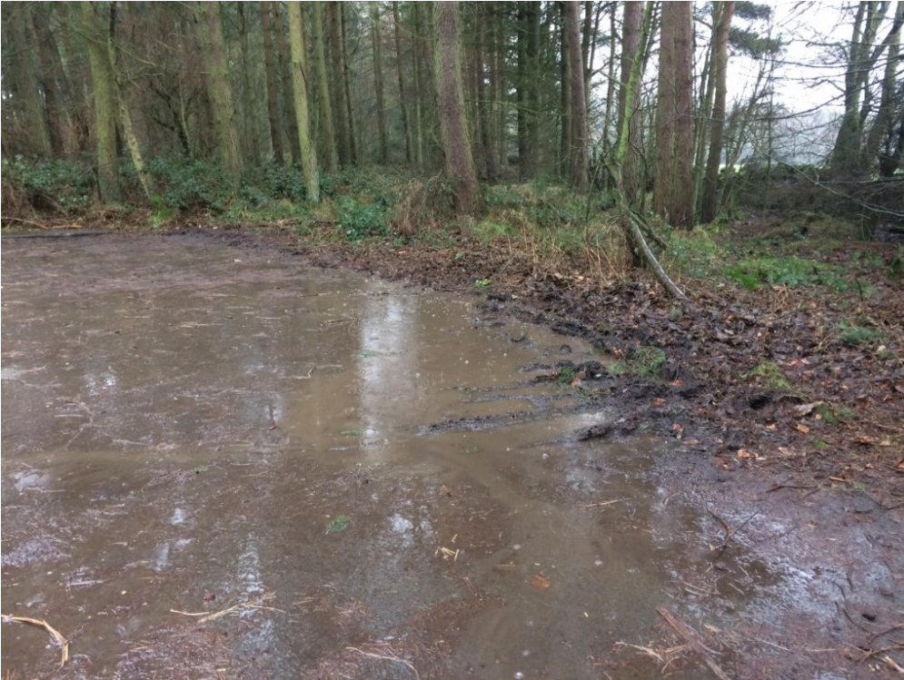
Figure 1 Surface and drain cleaning, edging and full bay lining required
