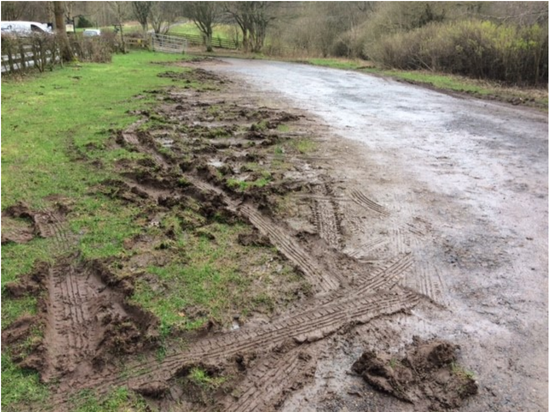
Figure 6 Overflow area acquired in 2019, unusable in wet conditions due to unbound surface
